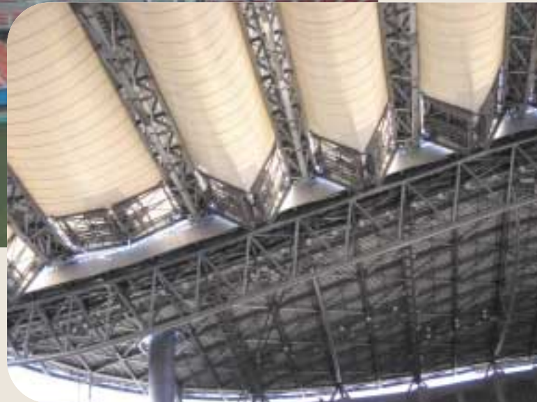
Kayaba's retractable roof system, used in the Toyota Stadium
